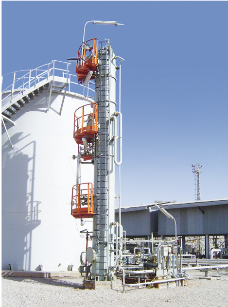
Vacuum Deaerator Package of Binak Desalting Plant
