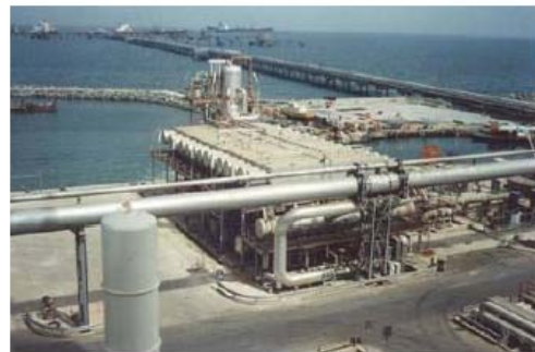
MSF desalination Plant
